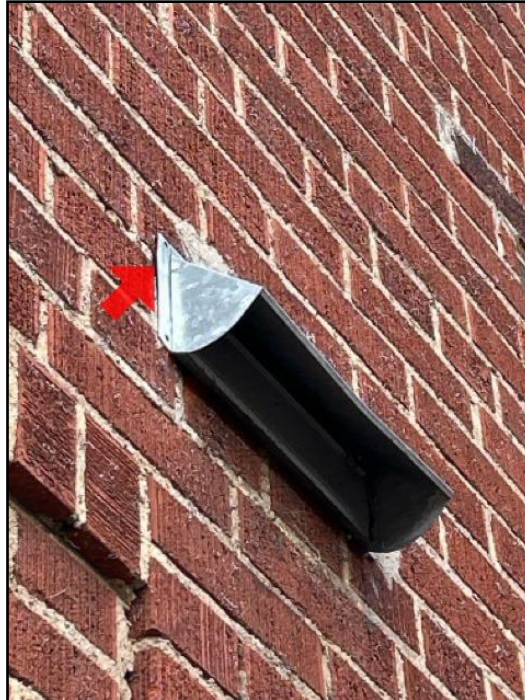
Caulking deteriorated/missing
