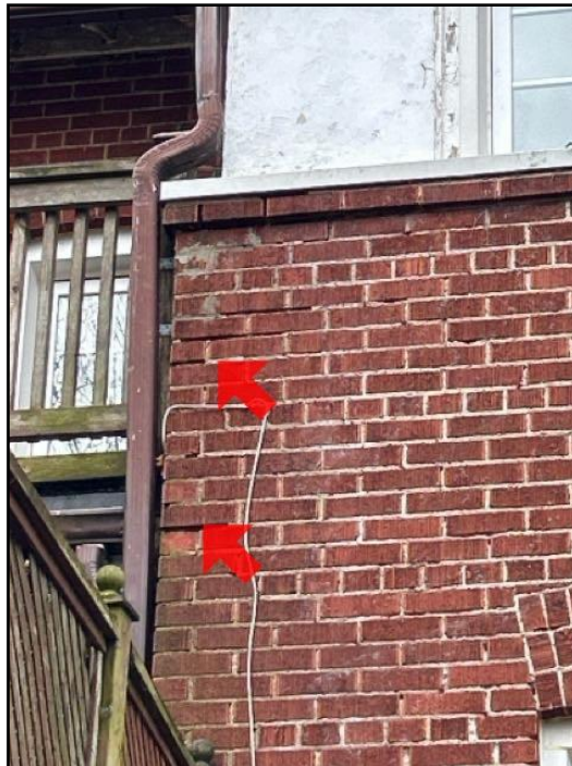
Mortar deterioration
