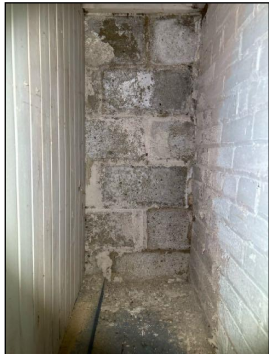
Efflorescence
