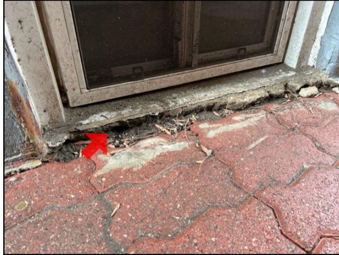
Sill deteriorated
