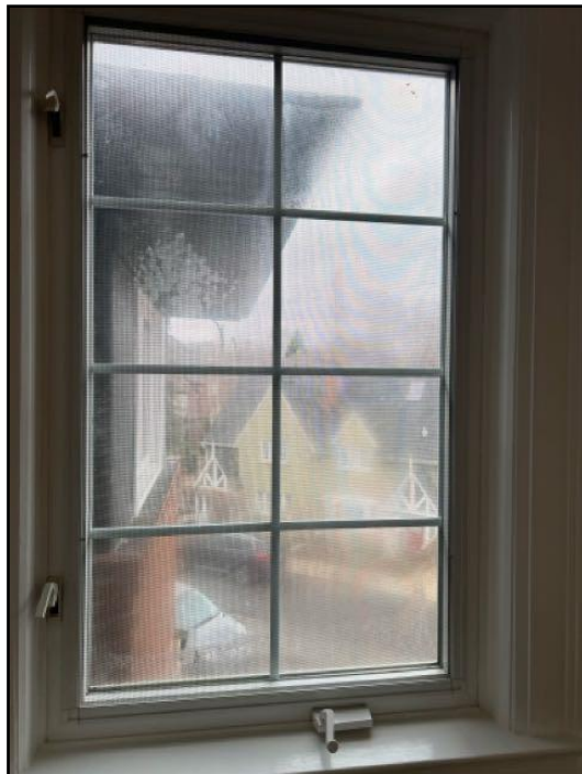
Lost seal on double or triple glazing...
