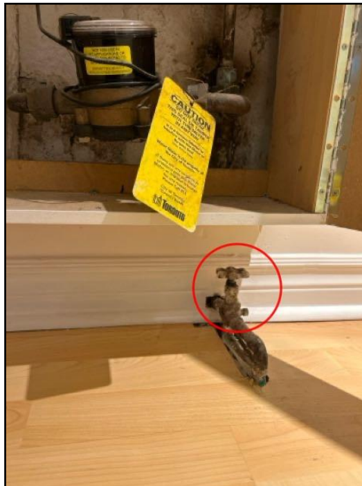
Front of the basement
