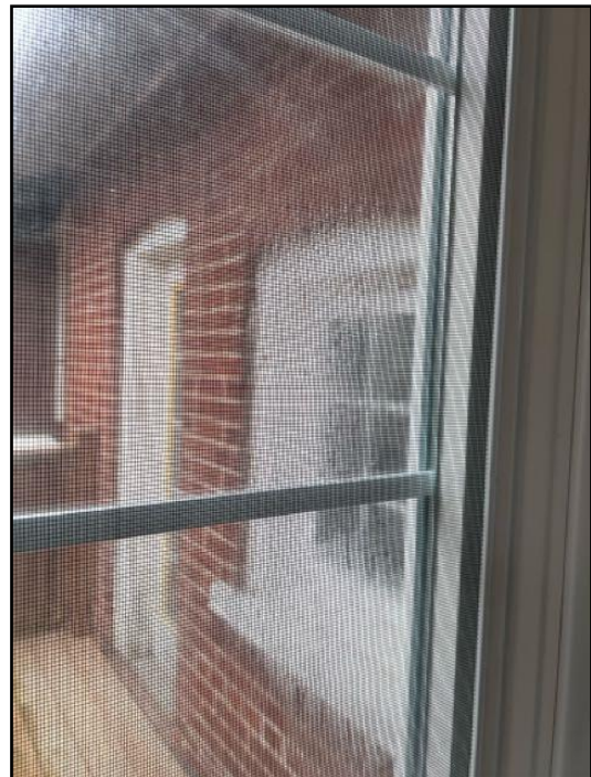
Lost seal on double or triple glazing...
