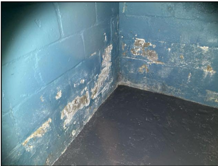
Efflorescence
